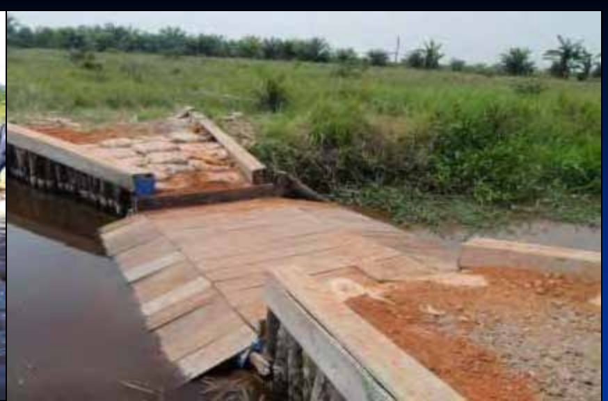
Canal block constructed by local communities.
