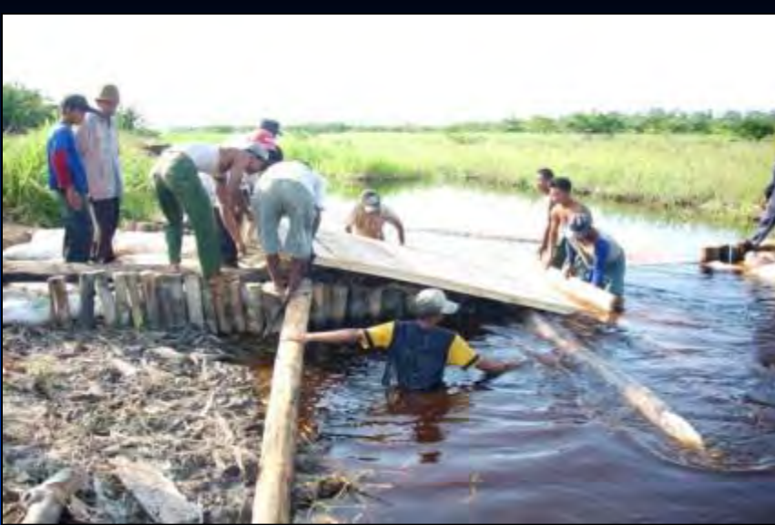
Canal block constructed by local communities.
