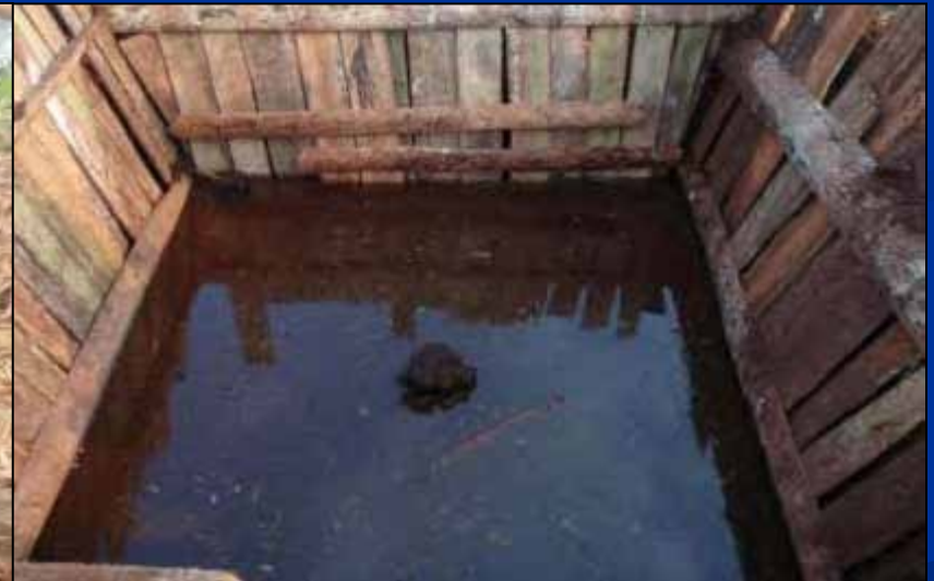
Canal block constructed by local communities.
