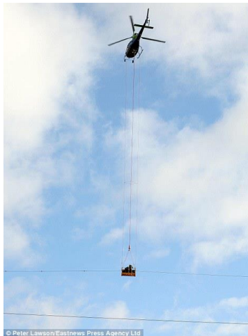
The Use of helicopter to translocate raw material
