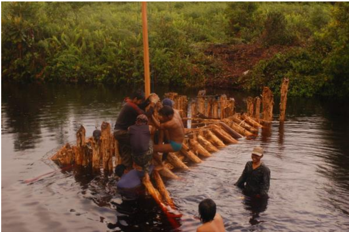
Manually building dams in a peatland drainage canal in Central Kalimantan, Indonesia. Photo: Hans Joosten.
